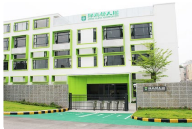
绿岛幼儿园 Green Island Kindergarten
